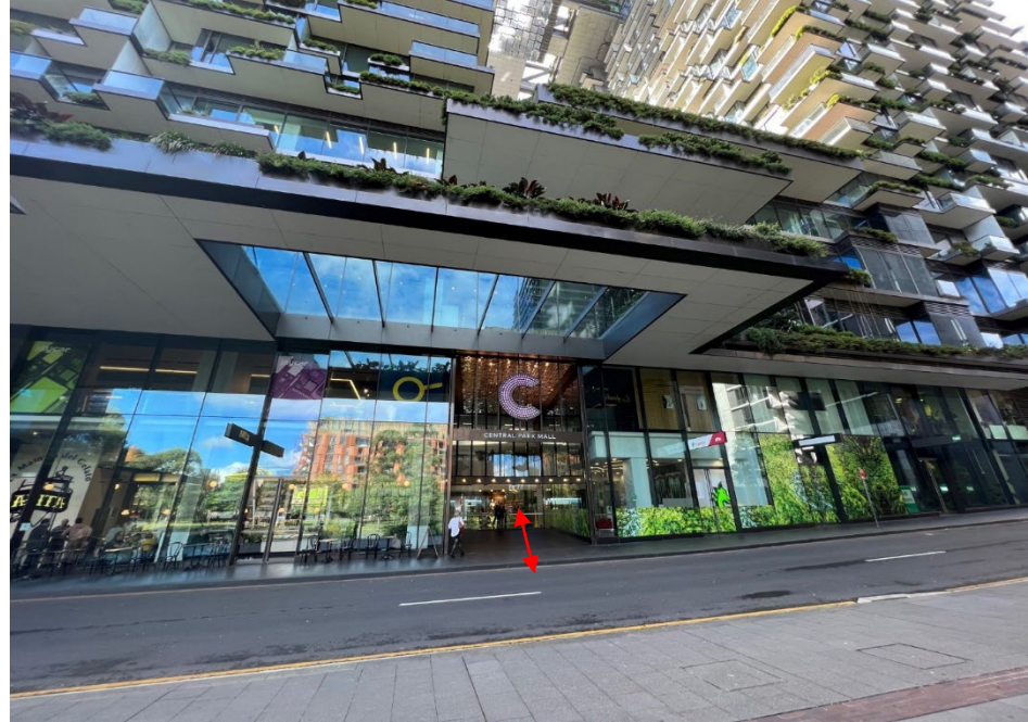
southern access at ground floor via Central Park Ave
