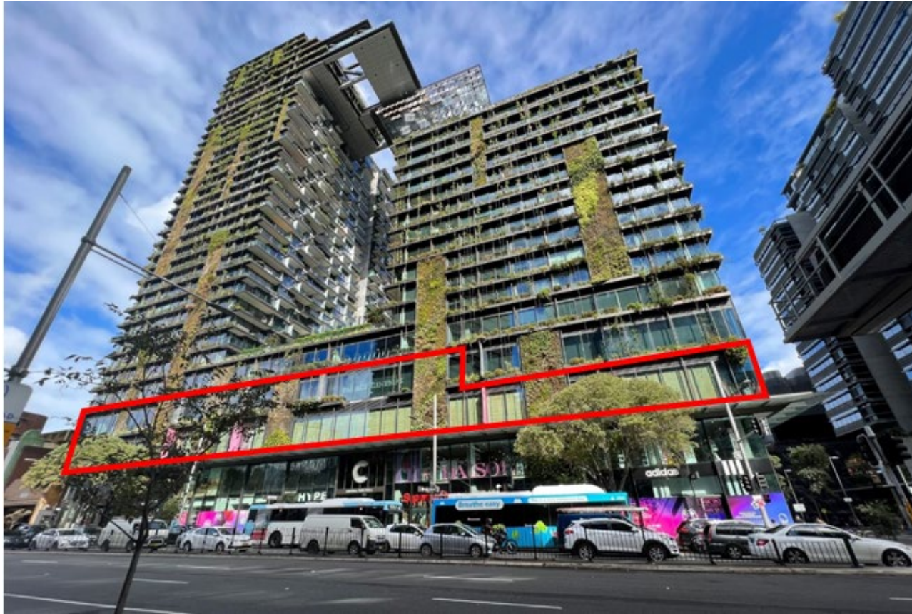
site viewed from Broadway looking south with Level 2 and Level 3 indicated in red
